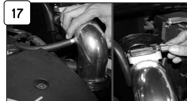
17 Install provided 5/8" hose to engine and tube. Reconnect MAF sensor harness. Reconnect battery terminals.
