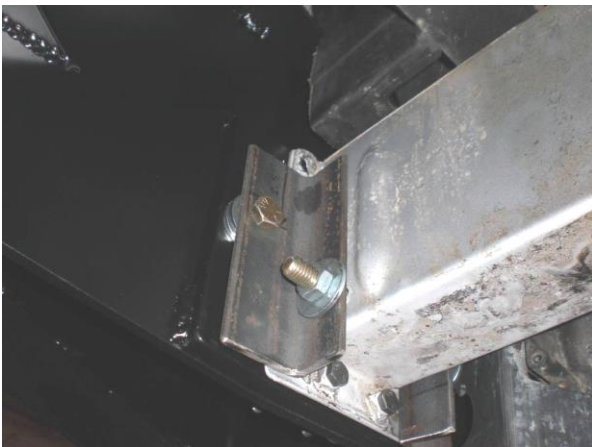
Figure 20: Steel support brackets bolted to frame
