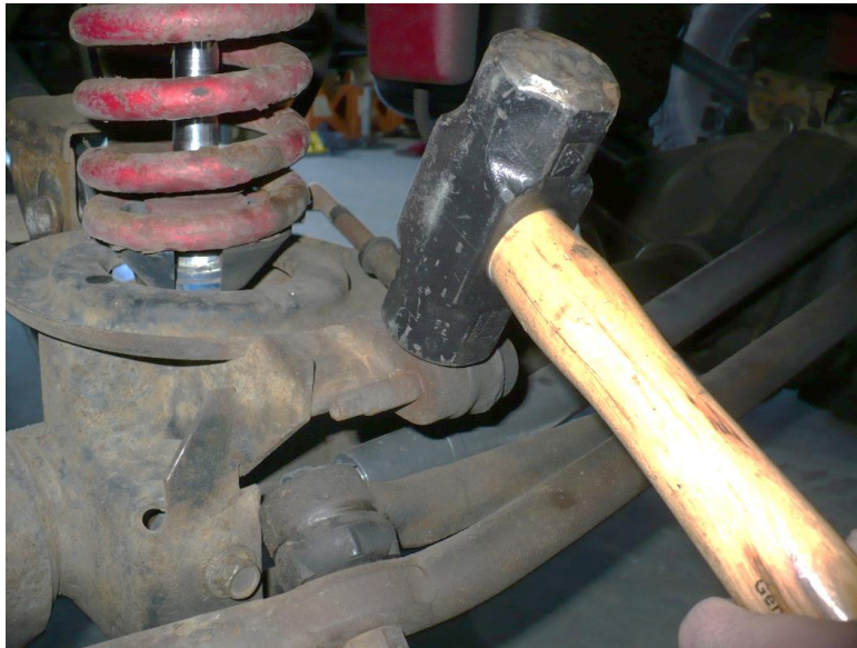
Figure 1. Using Hammer to Release Taper Fit
