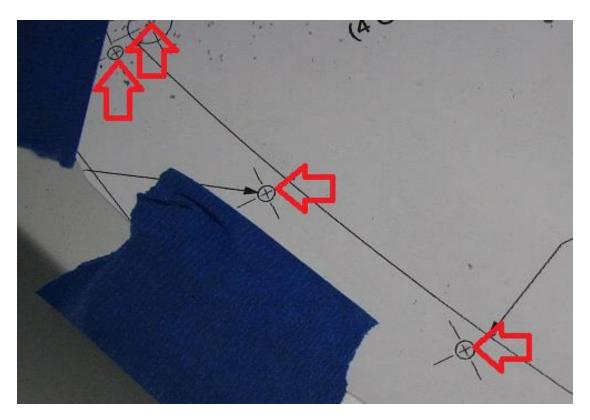
**2.15.** Using the smallest drill bit, 1/8", drill through the hood as shown below. Use high speed and light pressure to not break the bit or go plummeting through the hood and scratching it.
