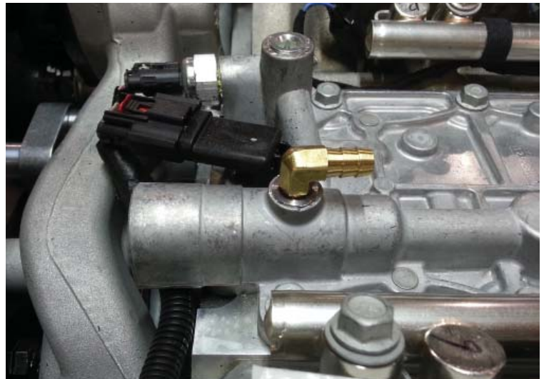
Barb Fitting Installed In Valley Cover
