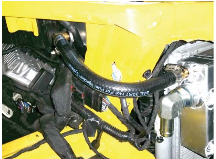
Fill Tank Hose Connected
