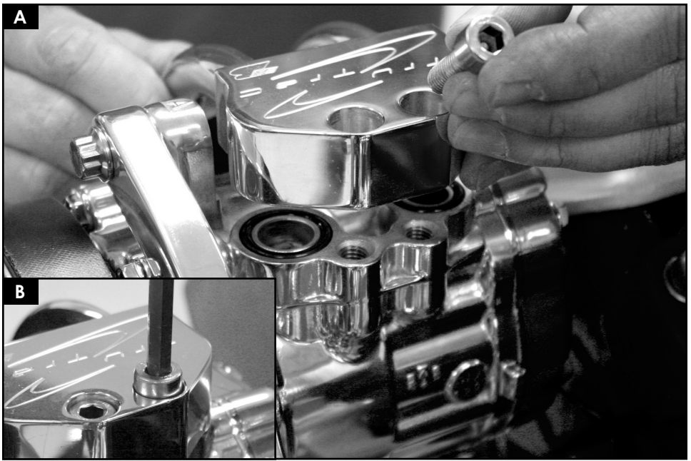
Figure 16: Install Compressor Manifold
